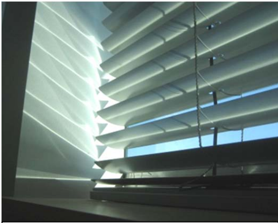
Advanced reflective blinds bounce sunlight up to the ceiling.
